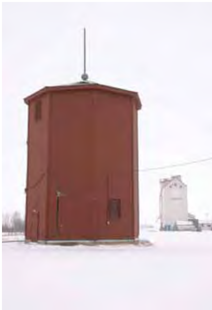
Completed in 1904, the tall wood frame Clearwater Canadian Pacific Railway Water Tower in Manitoba is an excellent example of an intact railway water tower. Twelve thick timbers are set on concrete bases and are strengthened with cross-braces that support the cedar-lined water tank, which occupies the top half of the structure. The water tower retains many of the original pipes, valves and controls used in filling and using the tank. When ceasing operation at a work such as this, the character defining pipes, valves and controls should continue to be subjected to regular maintenance to prevent their deterioration.
