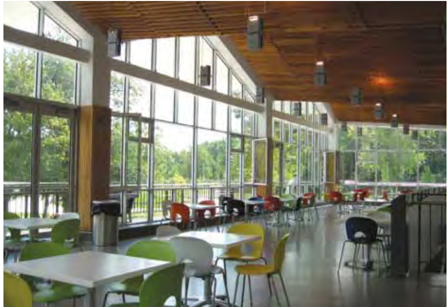
Wood was often used in modern buildings as a finish to contrast with more industrial materials, or as part of an acoustical treatment on ceilings and walls. The wood ceiling and column claddings of the Beaver Lake Pavilion in Montreal were carefully preserved as part of the recent rehabilitation of the pavilion.
