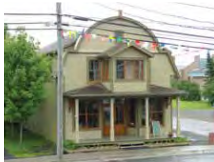
The Leopold Roy House in Saint-Quentin NB is a good example of a window, door and storefront restoration. Based on photographic and physical evidence, the original finishes and designs were uncovered and repaired or replaced in kind.
