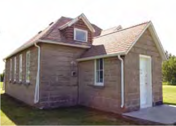
Tenby School in Lansdowne MB is a well-preserved and rare example of a village school built with concrete blocks, a material commonly used between 1890 and 1905 for homes and commercial buildings in southern Manitoba. The blocks were artfully formed on site by using three distinct moulds.
