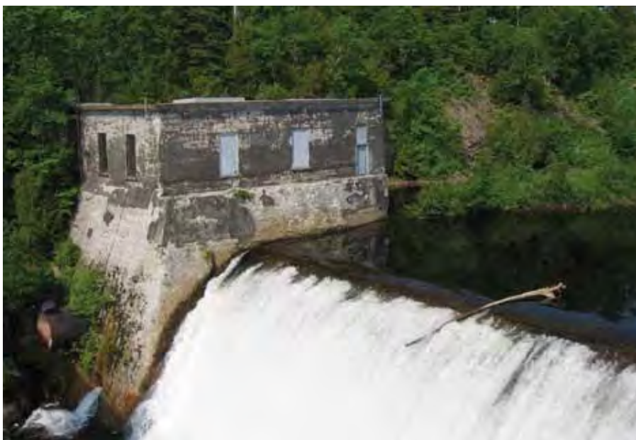
Remains of hydroelectric installations.
