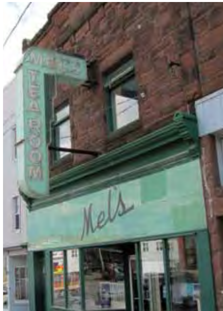
New signs (top right) should be compatible with the building in terms of size, scale, material, style and colour. They should also not obscure, damage or destroy character-defining elements. In some cases, as Mel's Tea Room in Sackville, NB (left), signs added later become character-defining elements in their own right. Character defining signage should also be maintained despite a change in use, such as this painted sign for the Hartt Boot and She Factory in Fredericton (bottom right), which has been converted into apartments.
