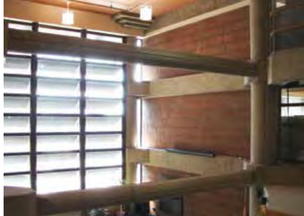
Using brick masonry in interiors is a long lasting, almost indestructible finish for public spaces. Brick walls and floors are character defining in many modern interiors such as the Joseph Shepard Building in Toronto. It is not recommended to apply paint or other coatings to masonry that has been historically unpainted or uncoated.
