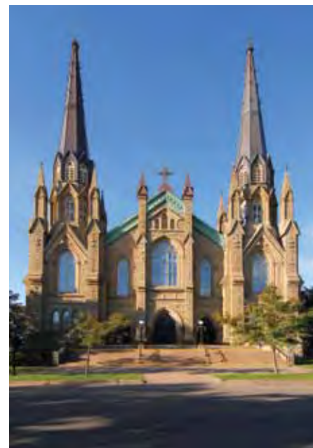
It is important to consider the expected life span of all elements that make up a roof assembly when repairing or replacing a roof such as this one on St. Dunstan's Basilica in Prince Edward Island. Roofing materials, such as copper and slate, need to be matched with flashings of a similar life span.
