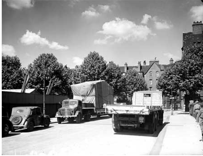
Figures 3.21, 3.22 & 3.23 Erecting an Aluminium prefab outside the Tate Gallery, London, 1945
