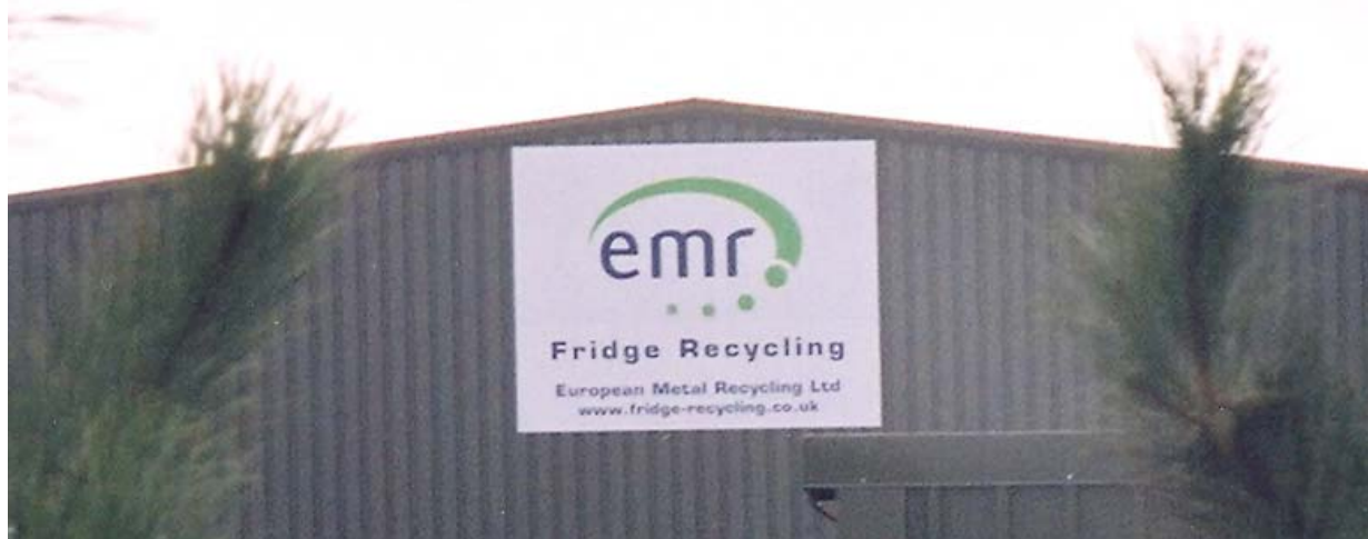
Figure 6.10 EMR’s Fridge Recycling facility in Willesden, London
