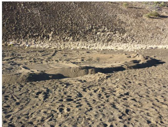
**Figure 6.4:** Landing pad berm constructed during the Mauna Kea deployment. Photograph courtesy of Kenneth Law.
