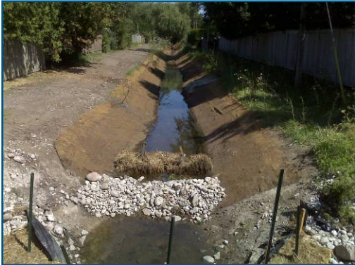
Sophia Creek – accumulated sediments were removed and stream banks were stabilized through native tree and shrub plantings.
