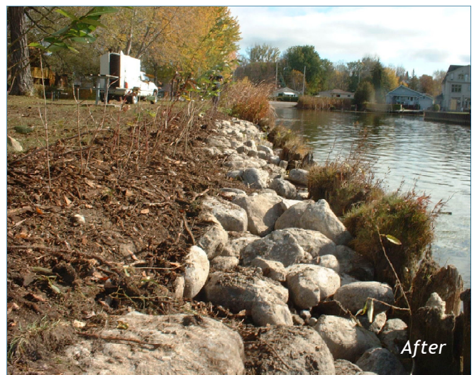
Walter Drive Erosion Control Project Before and After - approximately 630 m of shoreline was rehabilitated through bioengineering techniques including placement of river stone, fascines and live stakes, and the planting of 250 native trees and shrubs.
