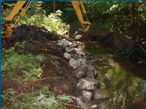
Bogart Creek – stream bed was enhanced through the installation of small boulders along the banks to promote fish habitat.
